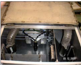
High pressure spray cleaning
